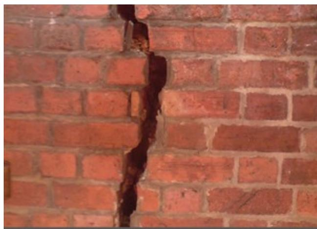
A 60mm wide crack, caused by settlement of foundations
